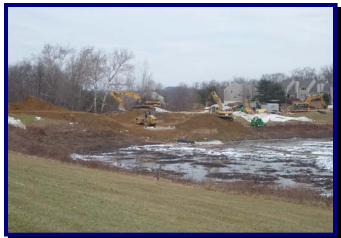
Dam restoration project managed by Hagerty personnel
